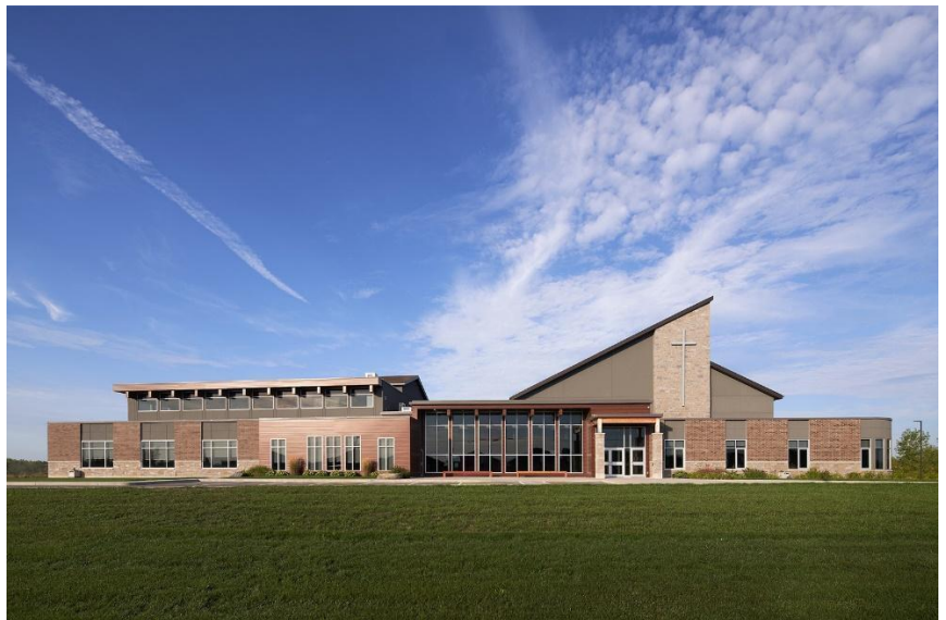
From the portfolio of the architects prior to the conversion: Trenton Wesleyan Church. source: https://arisearchitects.com/portfolio/trenton-wesleyan-church
